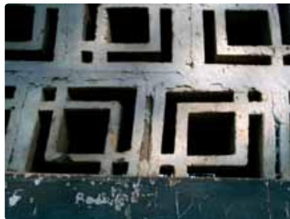
Photograph of a school window taken by Zambian school children (EENET)
